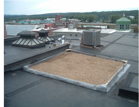
Rooftop nest patch in downtown Concord.
