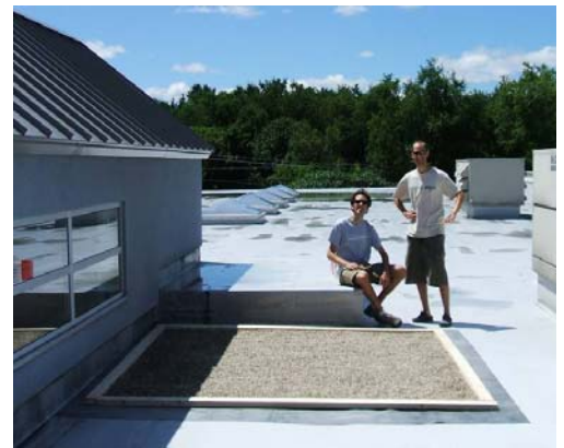
Completed nest patch. Photo by Ken Klapper.
