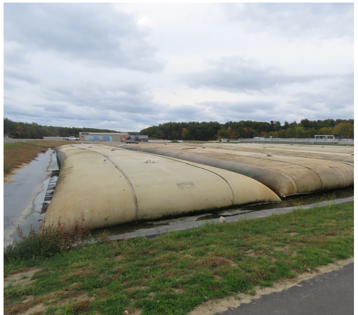
The construction at the Exeter WTP where Lagoon #4 used to be on 9-2-18 (top) and the “pillows” on 10-12-20 (bottom). Photos by Rebecca Suomala.
