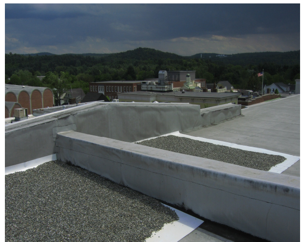
Two nest patches with white rubber membrane, 23 S. Main St., Hanover. Photo by Lou-Anne Conroy.
