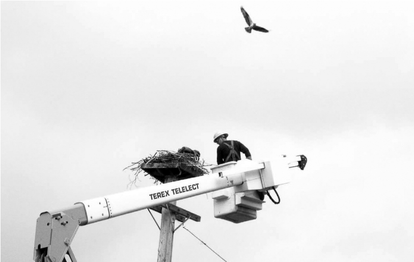
PSNH bucket truck helps get the job done while an adult Osprey keeps an eye on the chicks.
